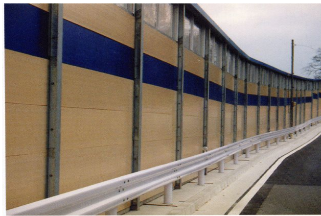
Highway Sound Barrier (TOMEI EXPRESSWAY)
